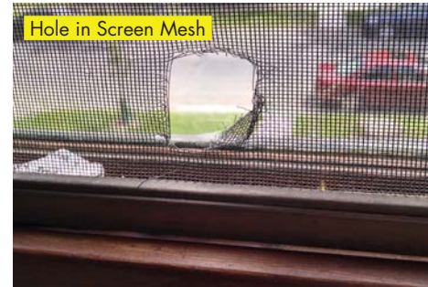
Improperly Installed Screen Mesh
